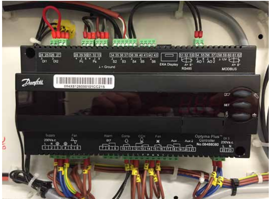
Picture1. Normal wiring
